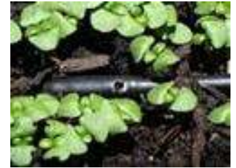
Irrigation – drip lines, sprinkler system
